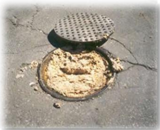
Sanitary Sewer overflows caused by fats, oils and grease.
