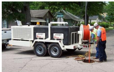
Lexington has to clean grease from lines to correct/prevent sewer overflows
